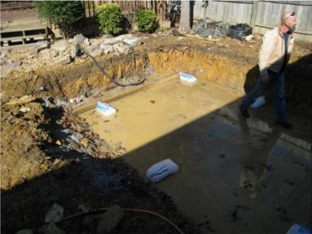
Figure 7. Ice Bag Positioning in Excavation
