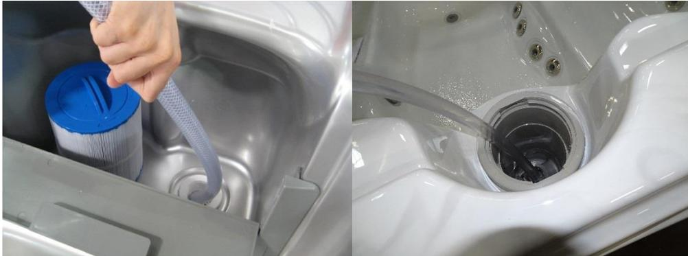
Figure 8. Filling Location in Filter Housing
