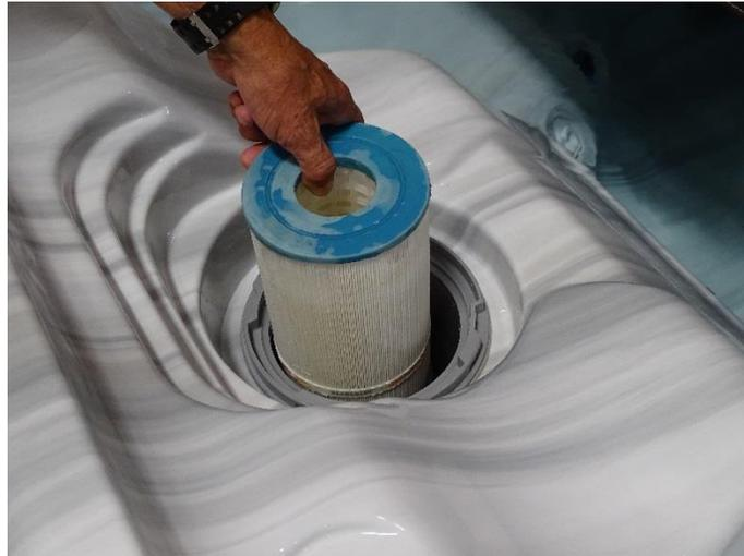
Figure 16. Drop in filter removal
