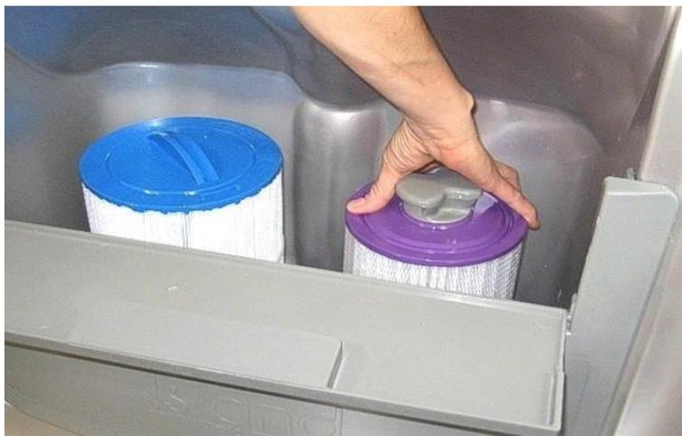
Figure 18. Screw-in Filter Removal
